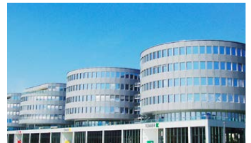
4 Towers, Steinhausen Production and assembly
